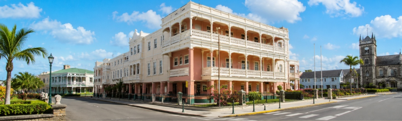
The National Assembly meets at Government Headquarters on Church Street, Basseterre, a building tied to the expansion of public administration in the mid-20th century. Its location anchors the Federation's legislature within the historic governmental centre of St. Kitts.
